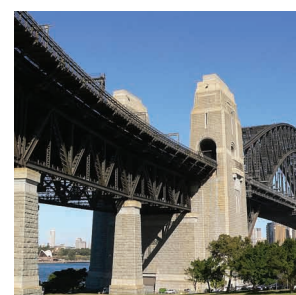
Sydney Harbour Bridge
