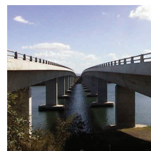
Taree Bridge Modular Expansion Joint Testing
