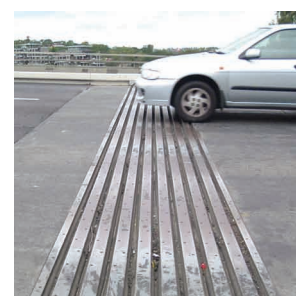
ANZAC Bridge Modular Expansion Joints
